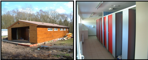
New toilet block nearing completion
